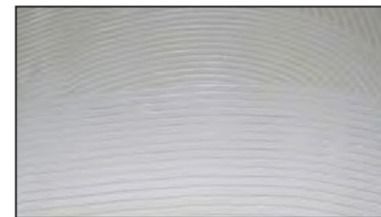
Example of properly troweled adhesive application
